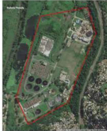
Northern Wastewater Treatment Plant, eThekweni Metropolitan Municipality, South Africa
